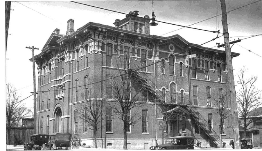
Christine School – 164 Market Avenue (Market & Third) Built 1872, last in operation 1963/64, demolished.
