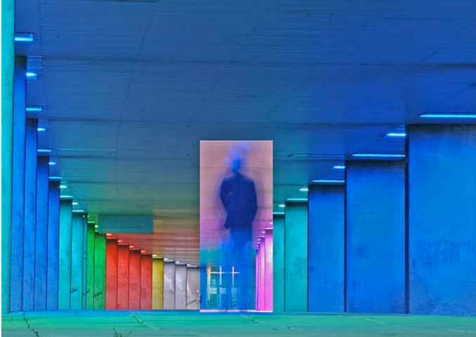
The underside of the Netherlands Center for Architecture (Rotterdam) suggests a possible decorative approach for Main Street beneath I-40.
